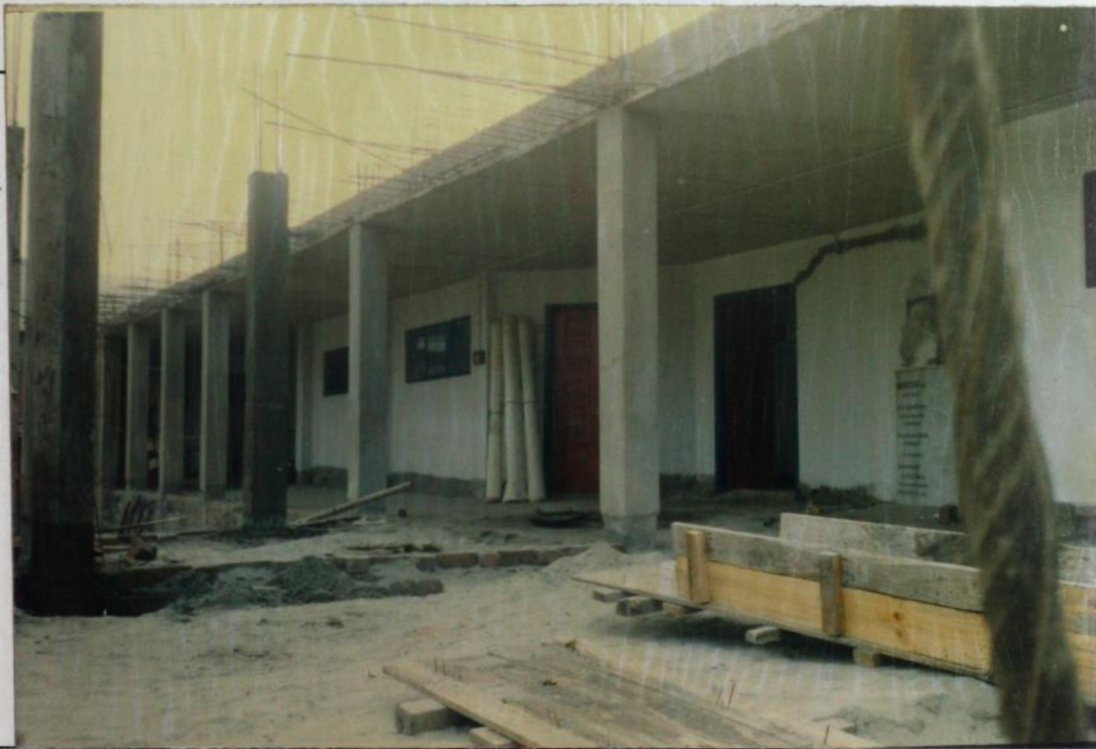
School building (Shishu Saroothi)
