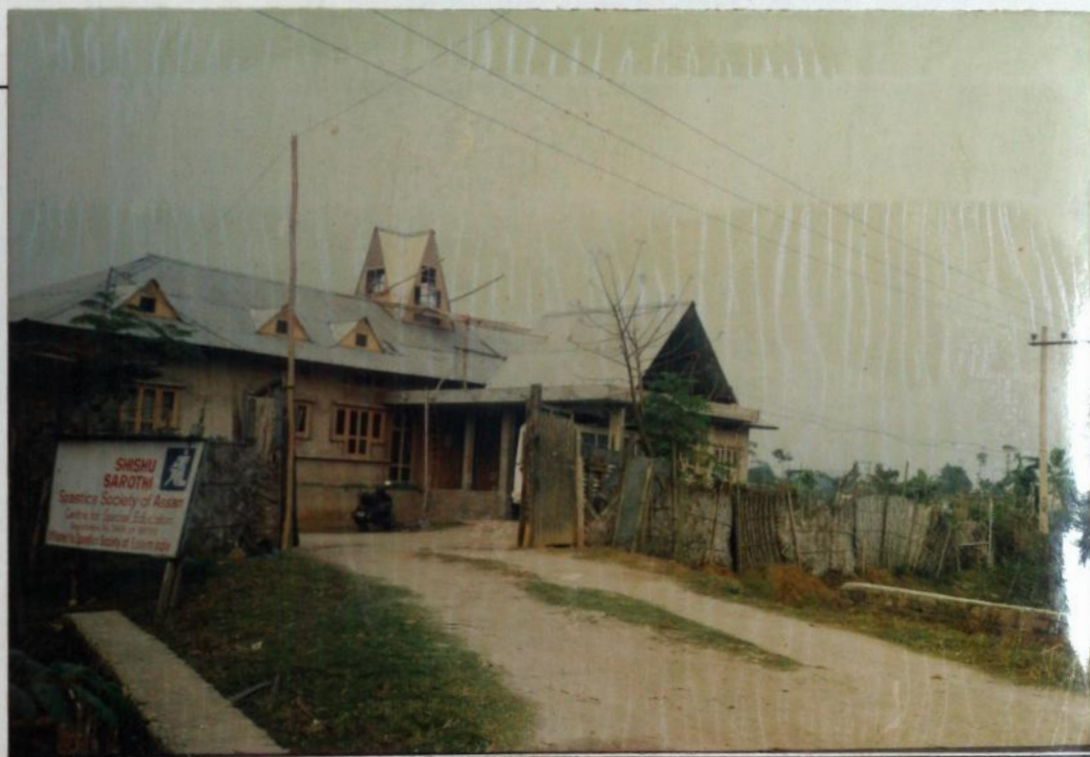
Shishu Sarothi (School building) located at Birubari, Ramkrishna Mission Road, Guwahati.
