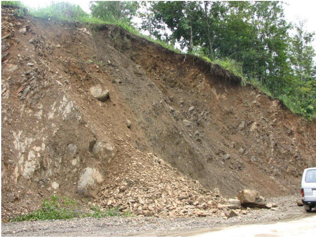
Plate 7.11a. Minor debris slide
