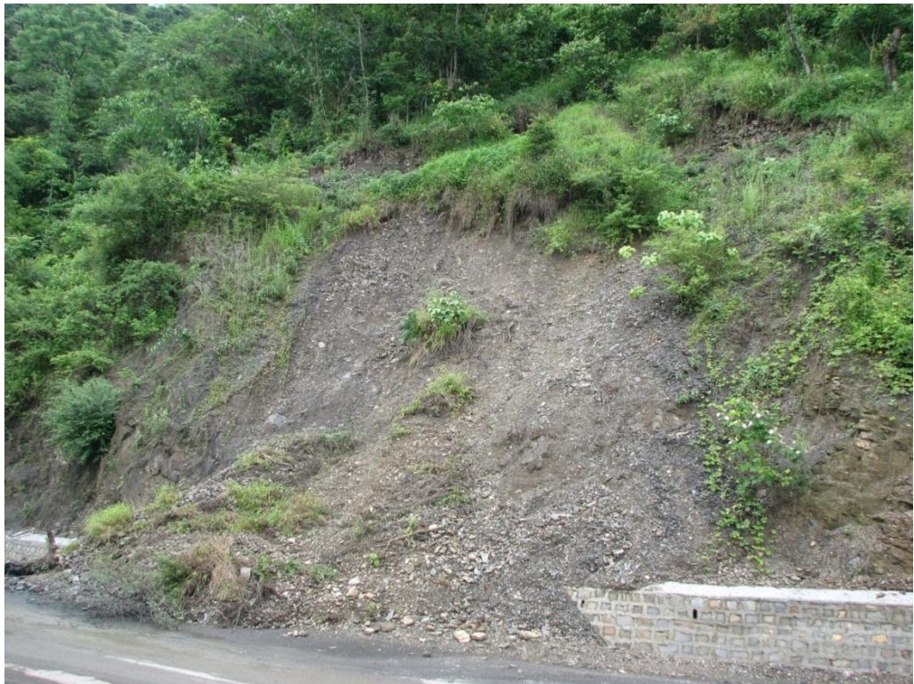
Plate 7.3b. Choked drain
