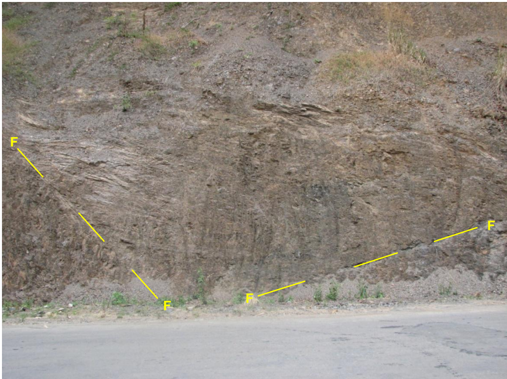
Plate 7.12b. Probability of wedge failure due to local faults
