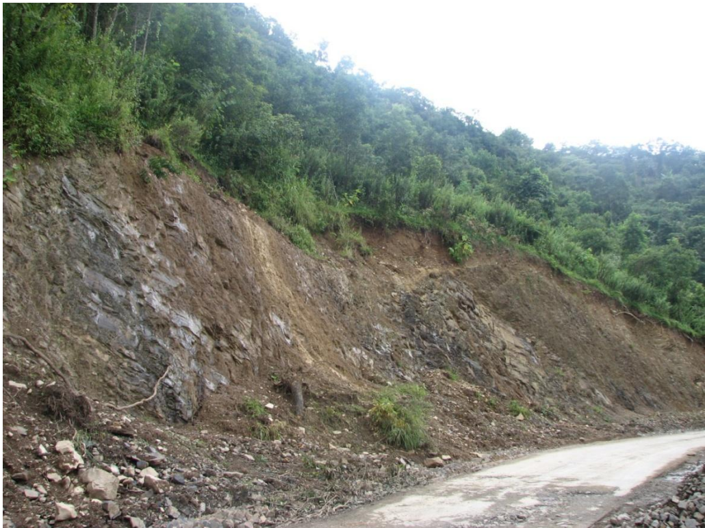
Plate 7.9b. Debris along the road section
