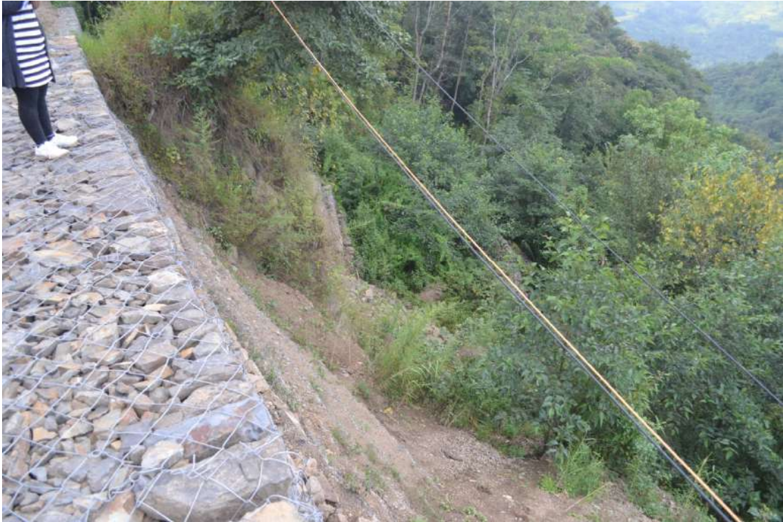
Plate 7.2.a Foundations of retaining wall on slide debris
