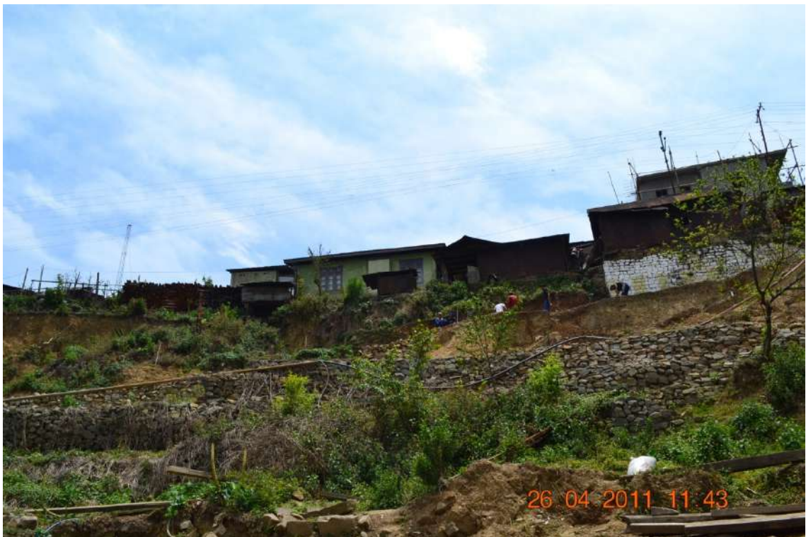
Plate 8.1.e Landslide inside the village
