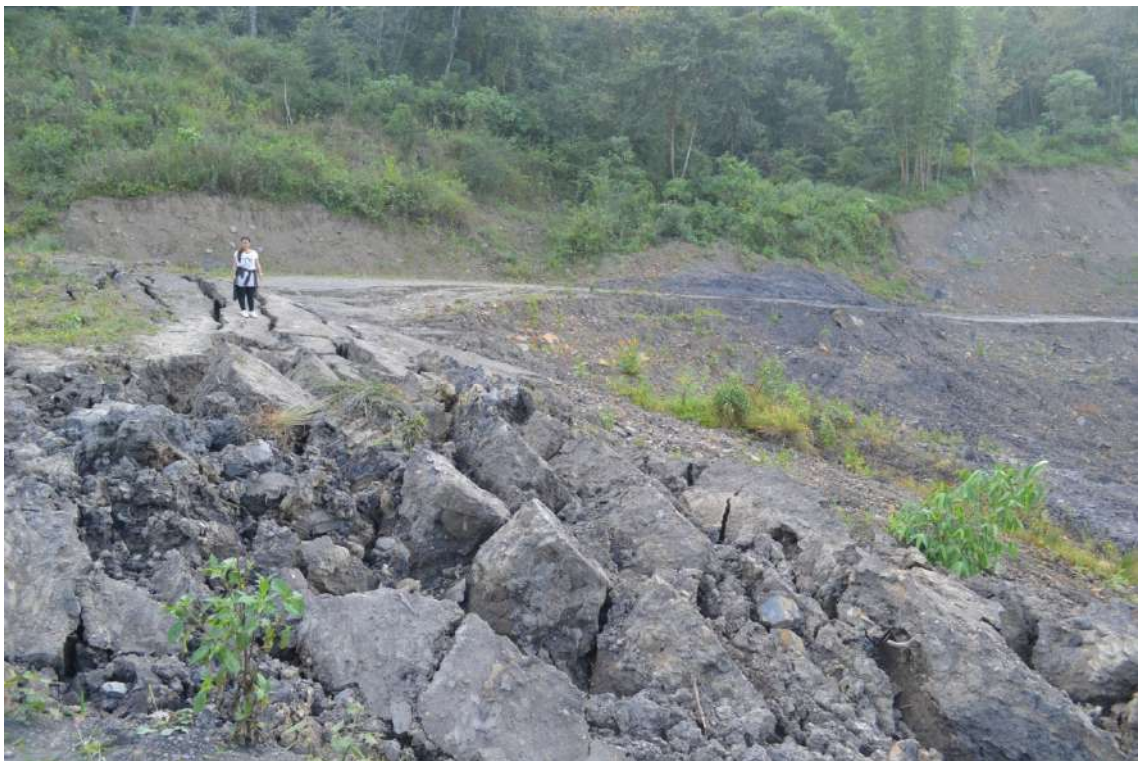
Plate 7.2.2.a Road section affected by landslide
