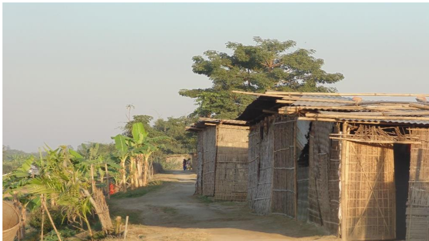
Plate 4.4: Land eroded people house on Embankment
