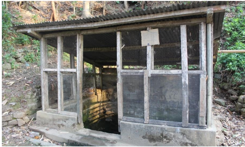
Village First Pond (Renovated and in use)
