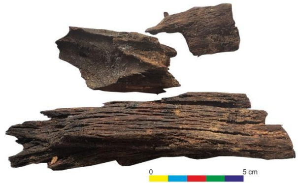
Figure 3.57: Decayed wood of Mhenkiton , Koro Old
