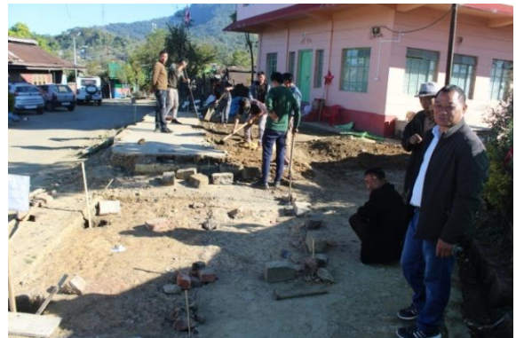
Figure 3.16b : Concrete floor debris is being removed
