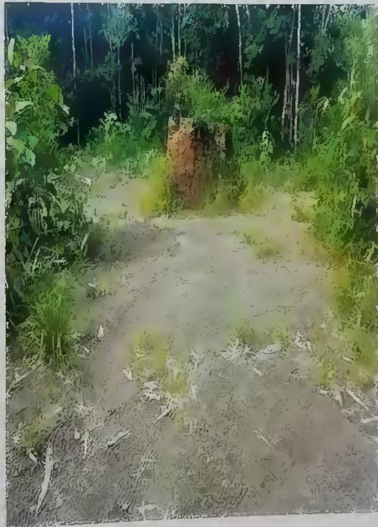
Plate : 4.17 Site for Electric Tower left abandoned
