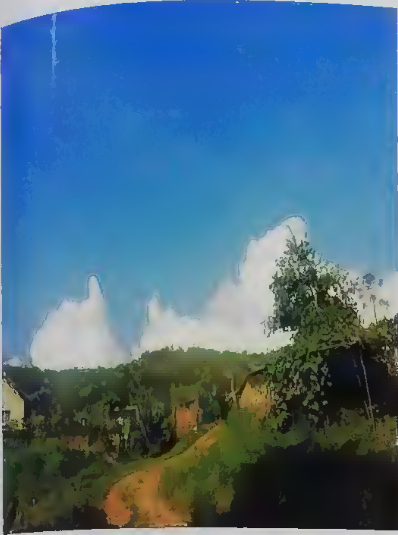
Plate : 4.14 Road without proper drainage
